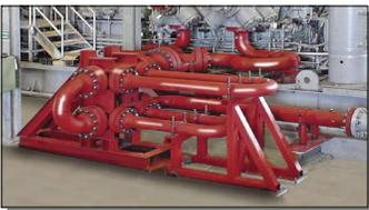
**1<sup>st</sup> Generation Field Test PAN on a Superior MH64 compressor**
